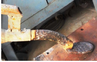
Fig Splash plate liquor gun nozzle model and its firing pattern in TNPL's recovery furnace
