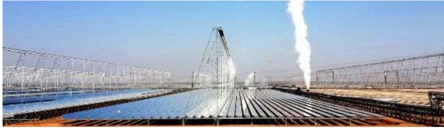
Dhursar (Rajasthan) 125 MW/ 2014
