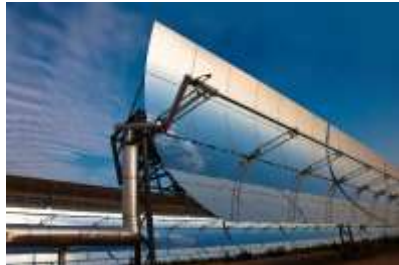
50 MW Godawari (Nokh), Rajasthan/ 2013
