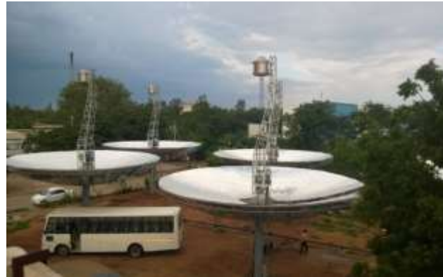
Paraboloid Dishes at Synthokem Pharmaceutical, Hyderabad (540 m 2 ; Process Heating)
