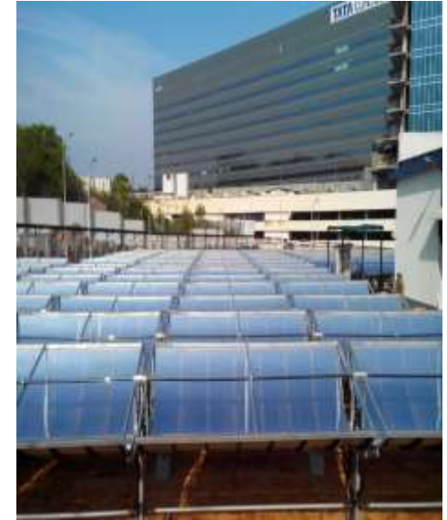
Parabolic Trough Collectors at Honeywell Technology Solutions, Hyderabad (820 m 2 ; Cooling)
