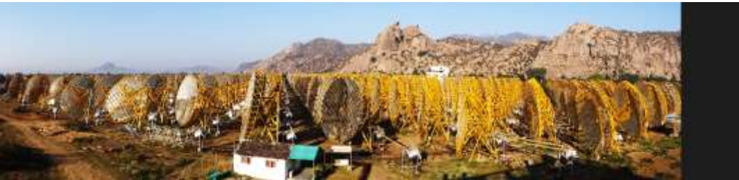
1 MW Mt. Abu, Rajasthan/ 2017
